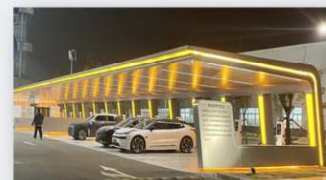
" wind-solar-ESS-charging " Comprehensive Energy Ecological Demonstration Station
