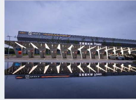
Geely Research Institute Wind-PV- ESS-Charging Demonstration Station
