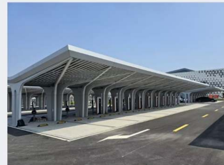
Quzhou Jidian PV-ESS-Charging Demonstration Station (V2G)
