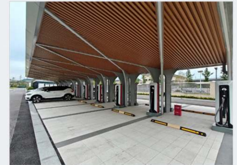
Hangzhou Jidian Storage-Charging Demonstration Station
